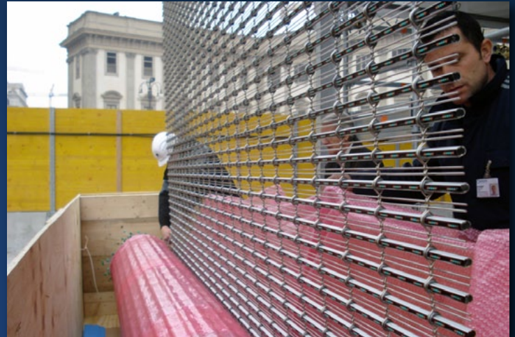
A Mediamesh panel being unrolled for an installation
