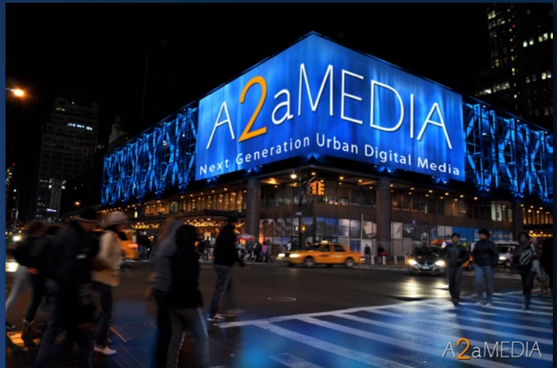
Port Authority Bus Terminal at 42nd Street and 8th Avenue
